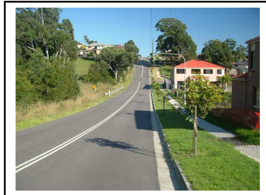
View West along Kings Avenue
