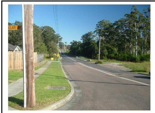
View west along Kings Avenue
